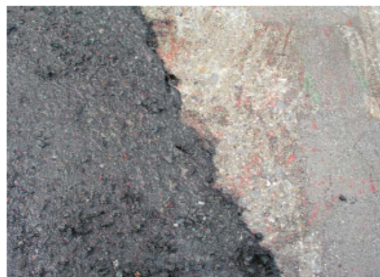
falch-nozzle technology uses 2500 bar and removes tar and resin without any problem
