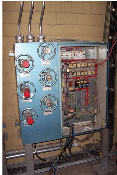
Conversion of control cabinet to 24 V
